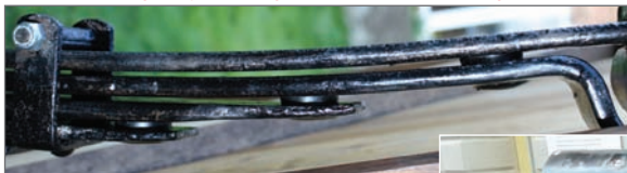
Photo 5: The assembled spring and rubber pads in position
