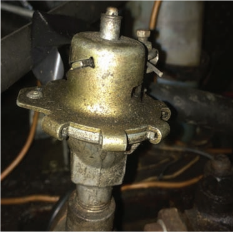
Picture 8. Heater valve
