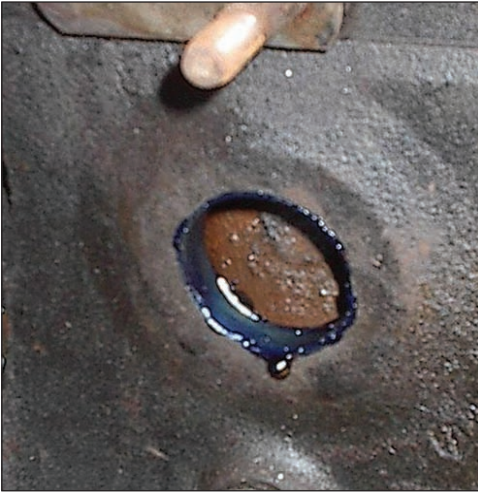
Picture 5 Core plug removed and sealant applied in hole.
